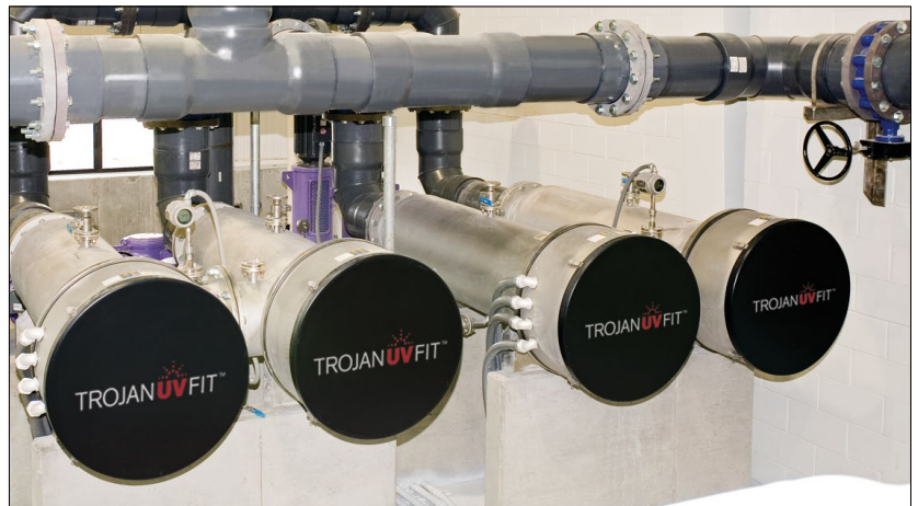
Chambers can be installed in parallel or in series for increased design and installation flexibility.
