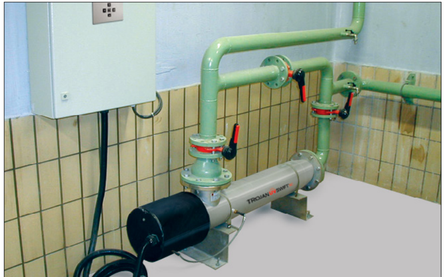
The highly efficient "L-shaped" design and low-pressure, high-output (LPHO) amalgam lamps result in an extremely compact footprint.
