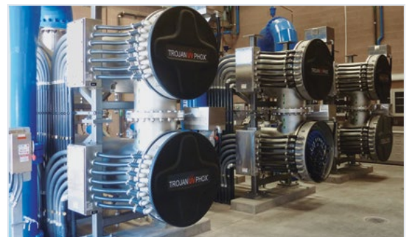
Figure 2. TrojanUVPhox ® system treating 1,4-dioxane
