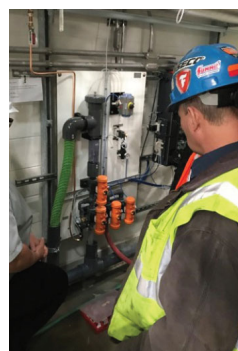
Figure 8. The EZ9130 sample preparation unit upfront the VFA analyzer
