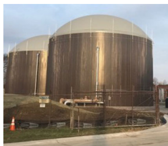
Figure 6. Anaerobic digesters at the Kenneth W. Hotz Water Reclamation Facility
