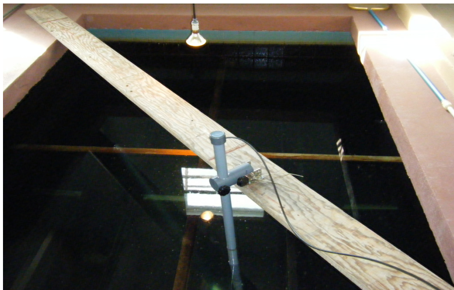
Figure 7. Solitax installation used for backwash study has been easily modified for long-term portable use at the Town of Bethlehem water treatment plant.
