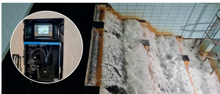
Cascade System - Drinking Water Production. Inset: EZ1000 Manganese Analyser in Drinking Water Plant
