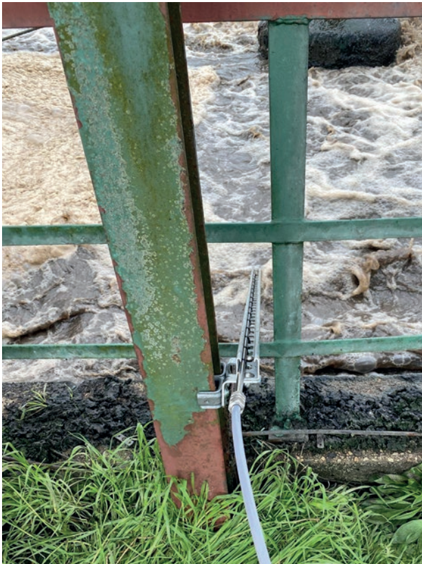
Sample line at the aeration tank
