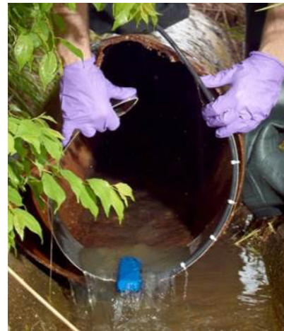
Hach sub AV sensor being installed in stormwater pipeline
