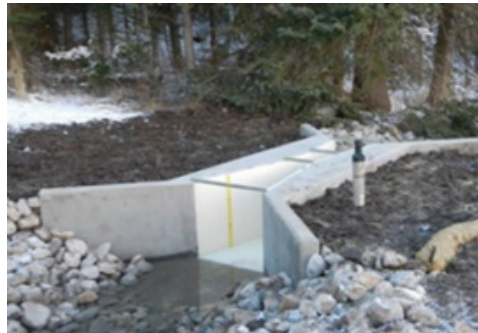
Parshall flume installation
