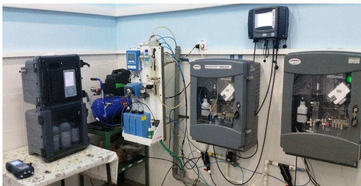
Figure 1 - Setup of the process analyzers at the DW plant. Service was running a verification test on AMTAX units at the time of the visit
