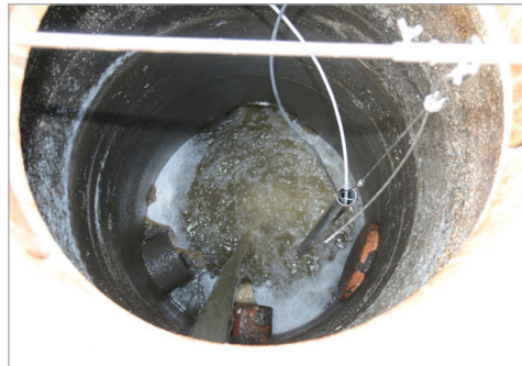
Figure 1. Inserting a liquid-phase sensor directly into the wastewater flow enables a more complete representation of the true concentration of H 2 S in that flow. This contrasts favorably against gas-phase-only sensors that can under-represent the scope of the problem based on the distance between the water and the sensor or the amount of turbulence in a wet well.
