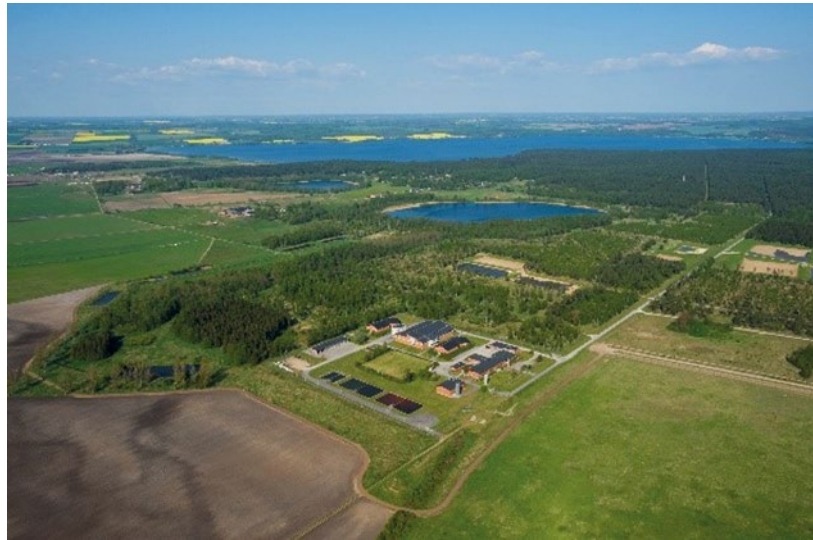
Aerial view of Vomb waterworks
