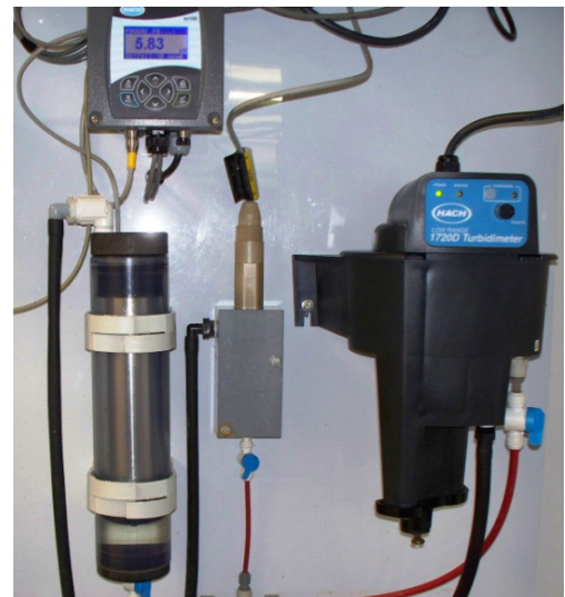
Figure 2: Raw water monitoring instrumentation at Soldier Canyon plant. Left: general view, right; LDO sensor in a flow cell, pH probe, and turbidimeter monitoring one sample stream)
