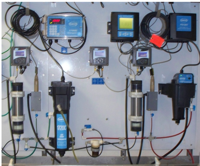
Figure 2: Raw water monitoring instrumentation at Soldier Canyon plant. Left: general view, right; LDO sensor in a flow cell, pH probe, and turbidimeter monitoring one sample stream)
