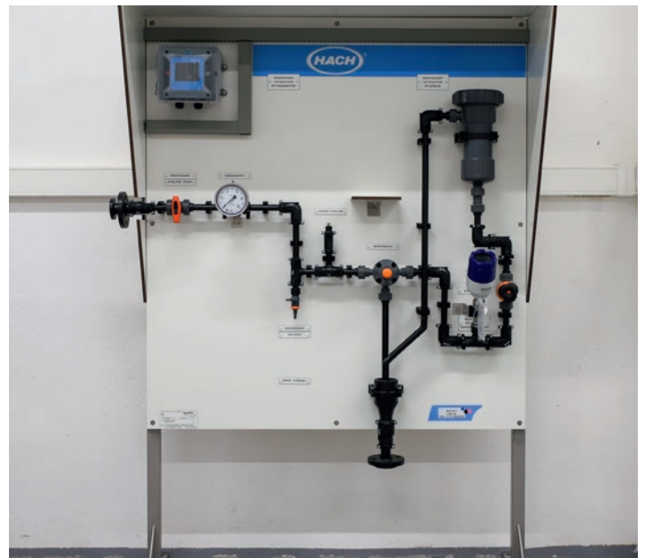
Anarack analyser rack for pH sensor
