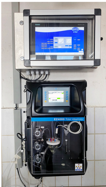
Figure 4: Industrial PC with ALK-RTC module and EZ4004 analyser
