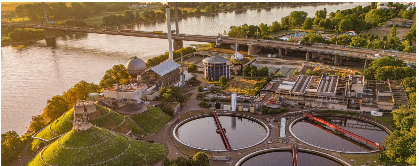
Figure 1: Aerial view of the Bonn-Salierweg wastewater treatment plant (Bildrecht Bundesstadt Bonn)
