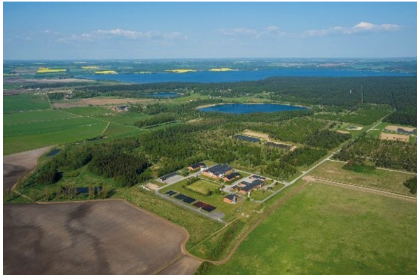
Aerial view of Vomb waterworks
