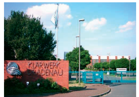
Picture 1: Hamburg WWTP
