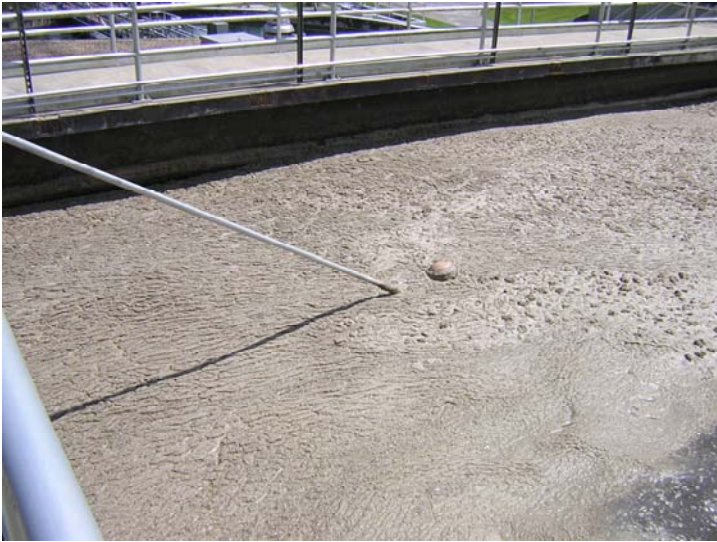
FIGURE 2: MEMBRANE PROBE IN GRU MAIN STREET PLANT'S ANOXIC BASIN.
