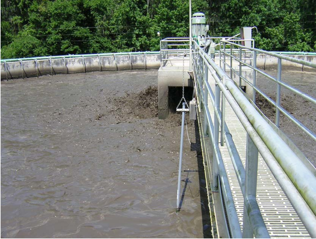
FIGURE 3: LDO PROBE IN A DIGESTER AT THE GRU MAIN STREET PLANT.
