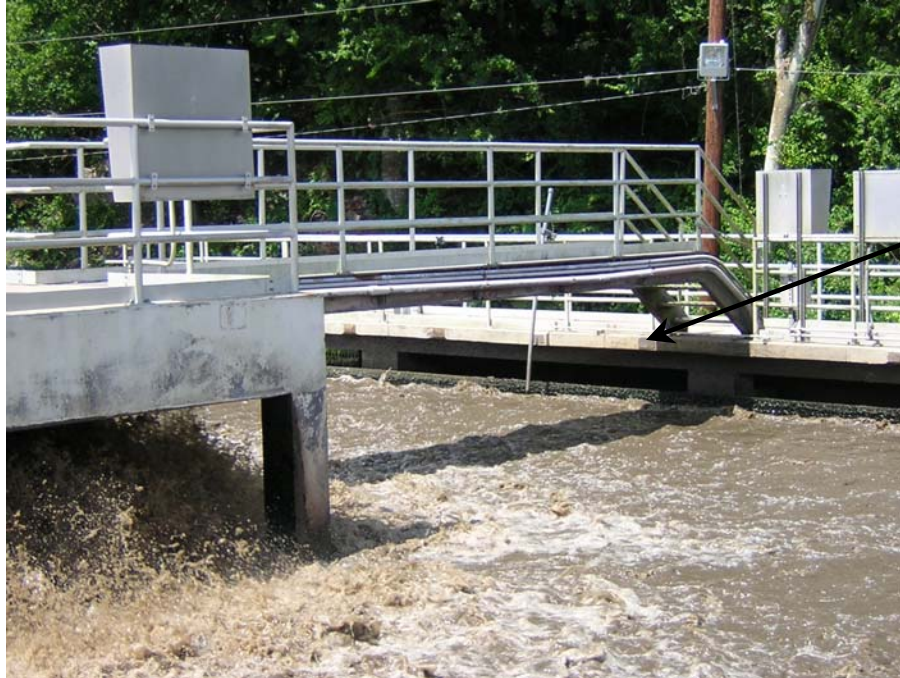
Figure 4: LDO probe in GRU Main Street Plant's aeration basin.
