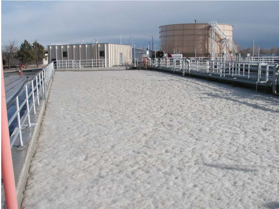
FIGURE 5: FOAM (APPROXIMATELY FIVE FEET) IN BASIN 1 IN LONGMONT
