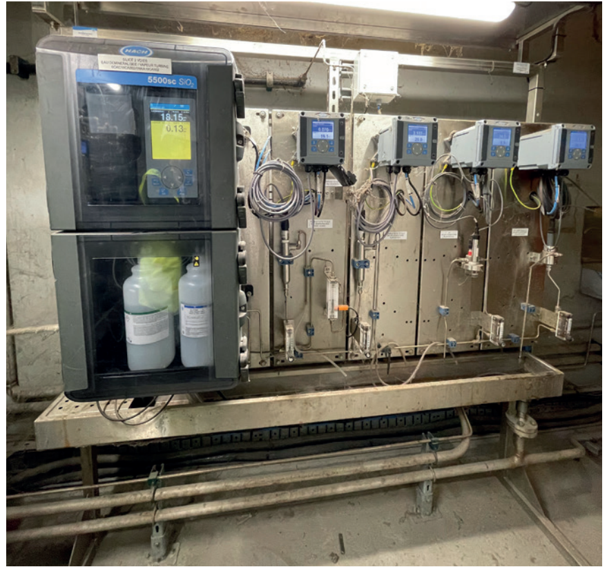
SWAS rack 2 with silica analyser, controllers, pH, conductivity, dissolved oxygen probes
