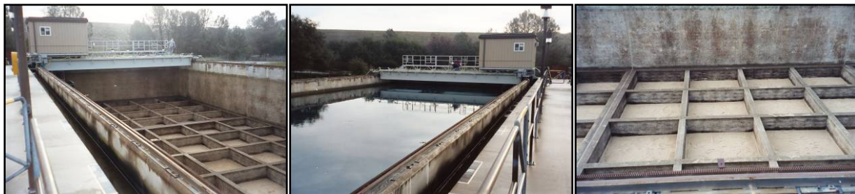
Figure 22: Traveling Bridge Filter
