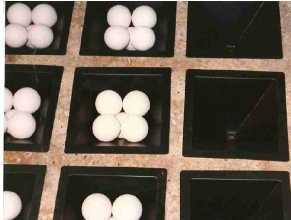
Figure 7: The Wheeler Filter Bottom
