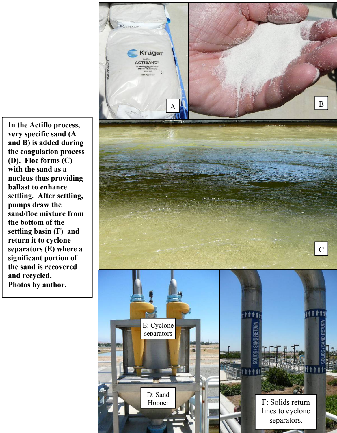
Figure 16: Actiflo process for ballasted flocculation
