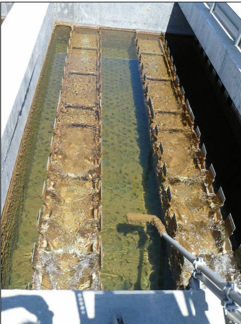
Figure 32: Tube Settlers enhance settling
