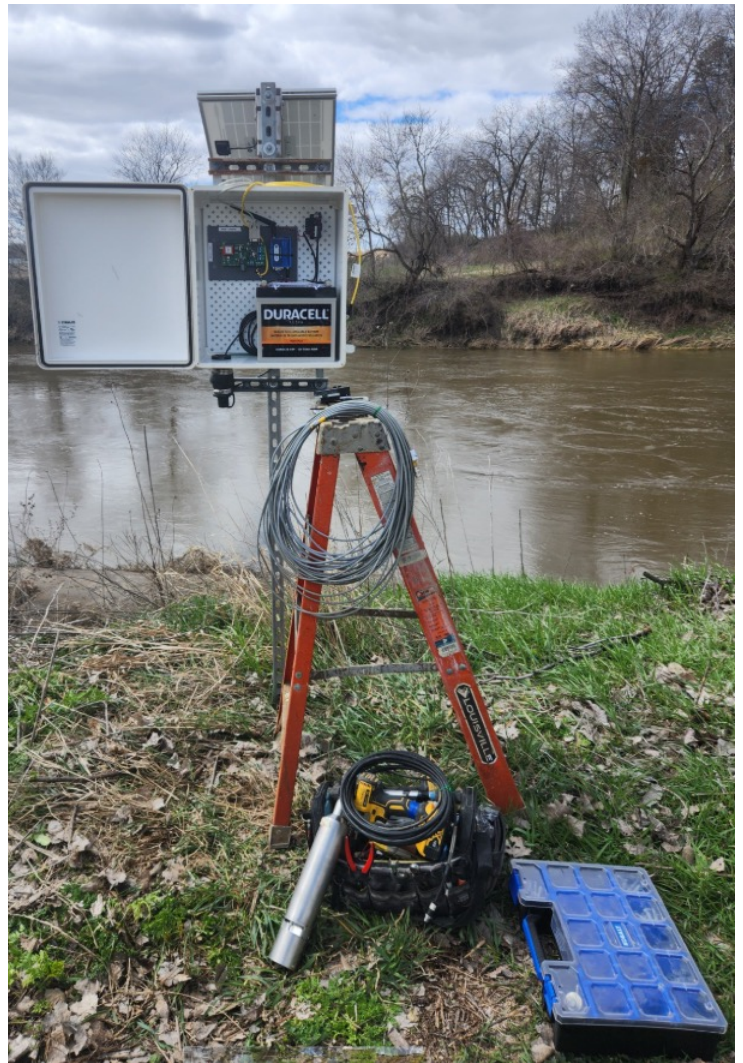
Photo 3: Depiction of an open monitoring station enclosure cabinet with photovoltaic solar panel, marine battery and portable NT3100sc nitrate sensor visible on the river bank, prior to seasonal deployment of a sensor in-situ. (Credit: IWQIS)
