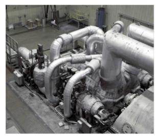
Monitoring of the entire steam-water circuits for both boilers is critical because the potential for condenser leaks can occur due to transient conditions at many locations via a variety of mechanisms. Conductivity is monitored on-line at seven different points for each boiler circuit: saturated steam; de-aerator; feedwater; boiler water; condensate intake and discharge; and re-heat steam. All but the boiler and condensate discharge monitoring points monitor cation conductivity.
