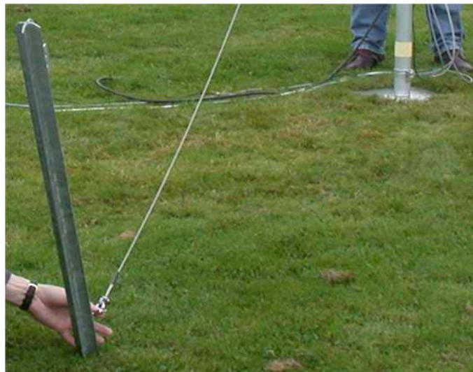
Figure 9: Determine the precise location of the nails using the guys.
