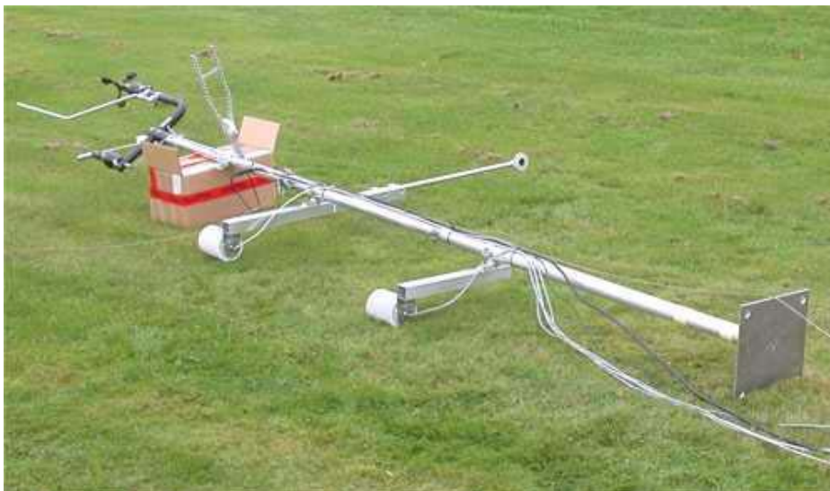
Figure 7: Mast, sensors, cables and guys are pre-assembled before the mast is erected.
