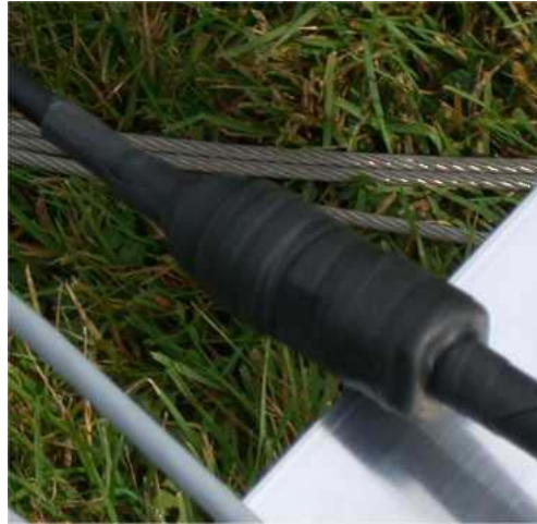
Figure 8: Protect all antenna connectors from water using self-amalgamating tape.
