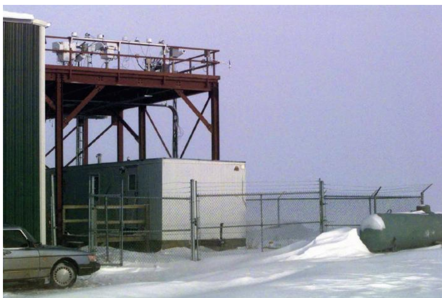
Figure 3.3. The support structure used to elevate instruments above the local horizon. The structural steel and concrete support structure at the Bratt's Lake Observatory, Meteorological Service of Canada.
