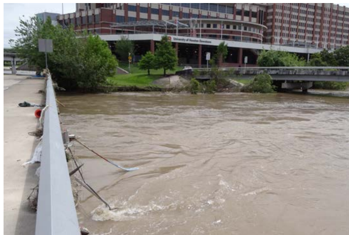
Radar mount struck by tree at Buffalo Bayou Downtown (Memorial Day 2015 Flood) (Photo courtesy of J. Lindner, Harris County Flood Control District)
