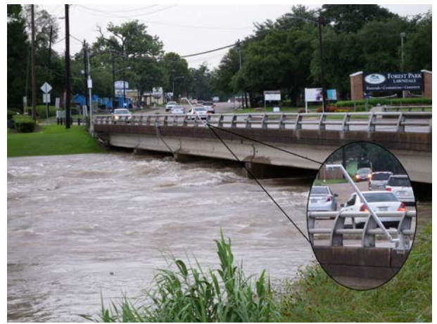
Brays Bayou at Lawndale Radar Unit (Memorial Day 2015 Flood) (Photo courtesy of J. Lindner, Harris County Flood Control District)
