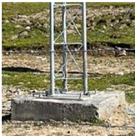
Figure 29. Examples of proper tower installation
