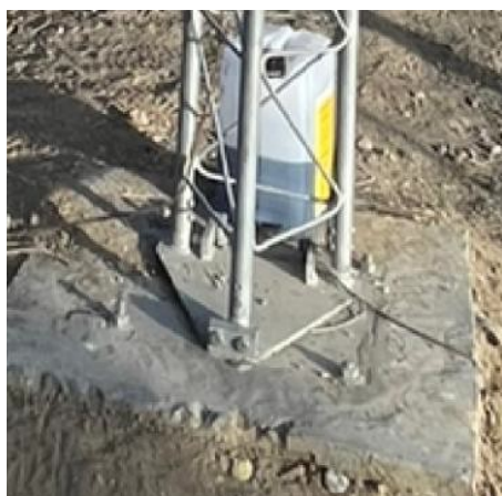
Figure 30. Examples of proper tower installation cont.
