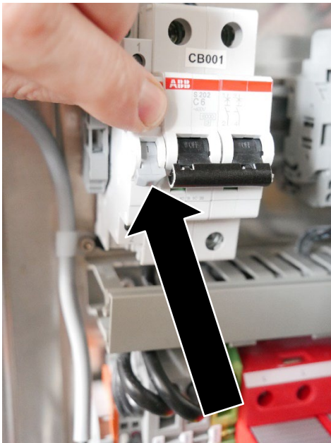
Figure 4: Switch position "UPS off"
