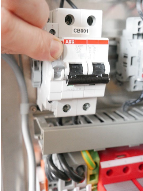
Figure 11: Switch position up for UPS on
