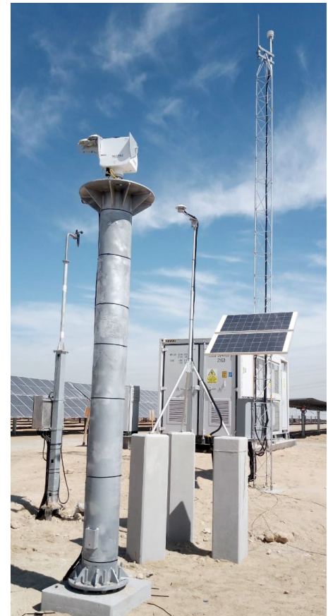
PV Met Station & Solys2 Sun Tracker at the Al Dhafrah Plant
